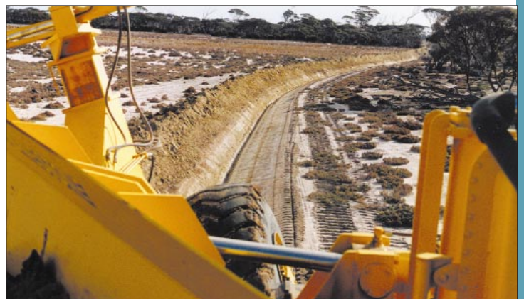
Digging a lateral drain
