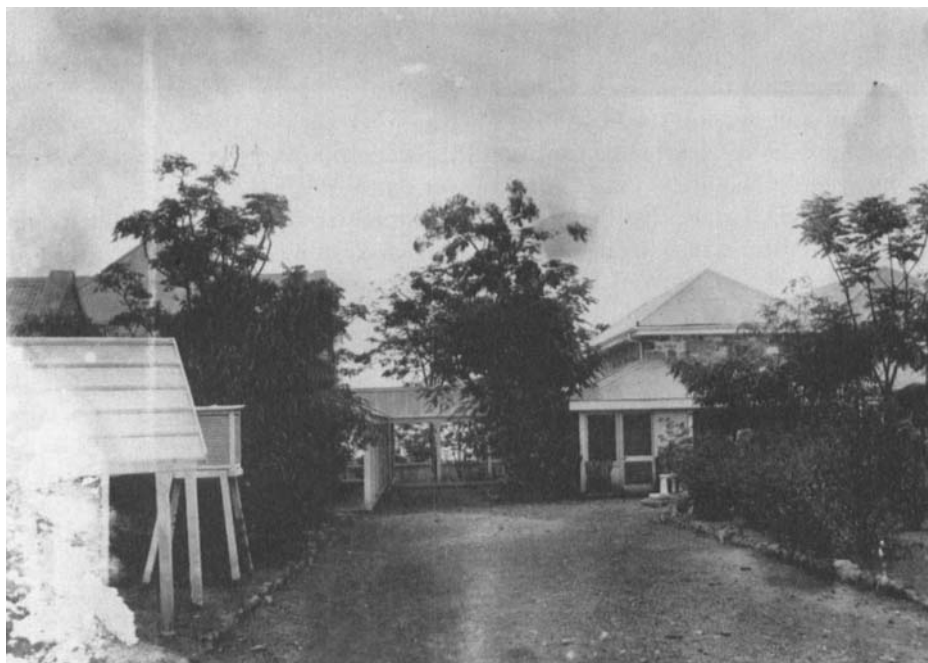
Figure 1. Stevenson Screen outside Darwin Post Office, 1890. Photograph 1/28 in the Tracey Collection, from the Northern Australian Collection of the State Library of the Northern Territory
